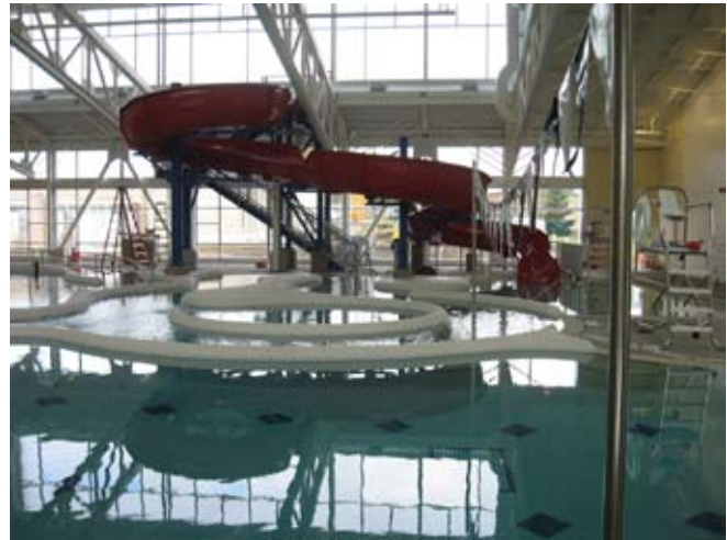
Technology will help a new Portland aquatic center save nearly 1.5 million gallons of water annually.
